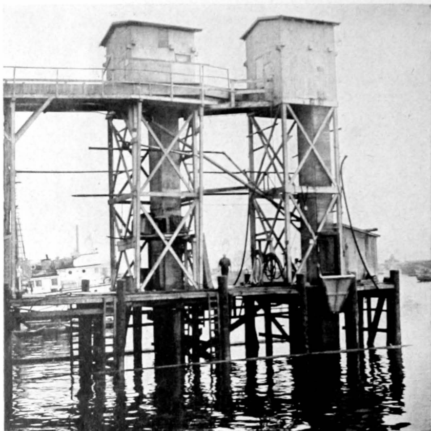
FIGURE 42.—Elevator and conveyor for unloading mackerel and sardine boats at Terminal Island, California.
